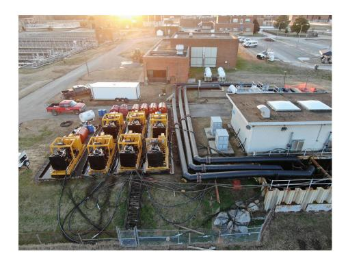
WMS performed 24/7 pump monitoring with onsite personnel and utilizing telemetry to ensure the successful operation of the equipment throughout the duration of the project.
